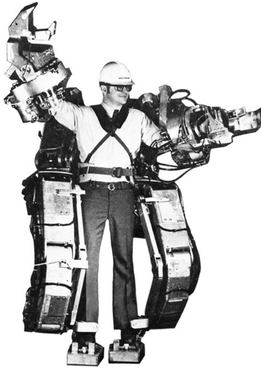
Figure 8: Hardiman from General Electric in 1965 was the first serious attempt to build a powered exoskeleton (“GE Report: The Story Behind the Real ‘Iron Man’ Suit,” n.d.).
